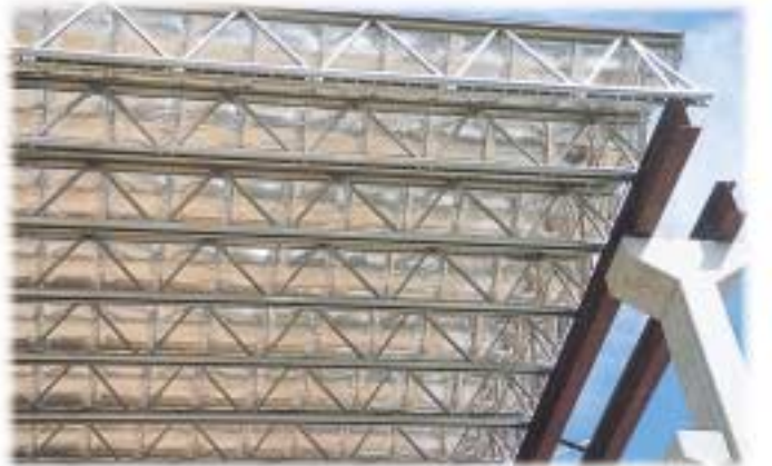
New Commercial Roof
